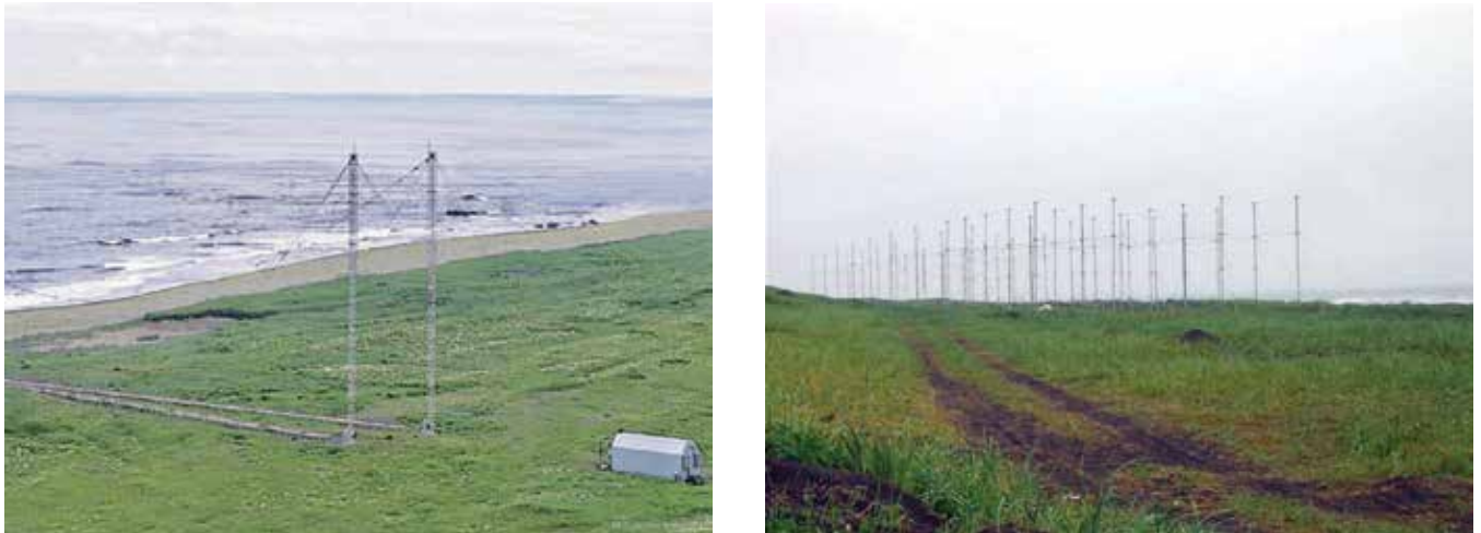
Figure 2: The Russian Podsolnukh (Sunflower) HFSWR is a large (1.5-km wide) shore-based HFSWR system featuring separate transmit (left) and receive (right) arrays that are usually positioned at least 1 km apart. | ROSOBORONEXPORT PHOTOS
